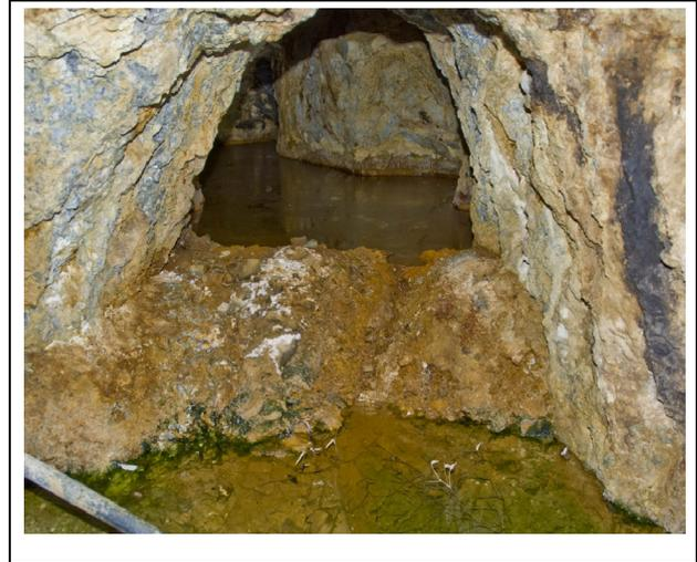
**Figure 5. North Percha Creek mine berm with formation of efflorescent crusts.**
